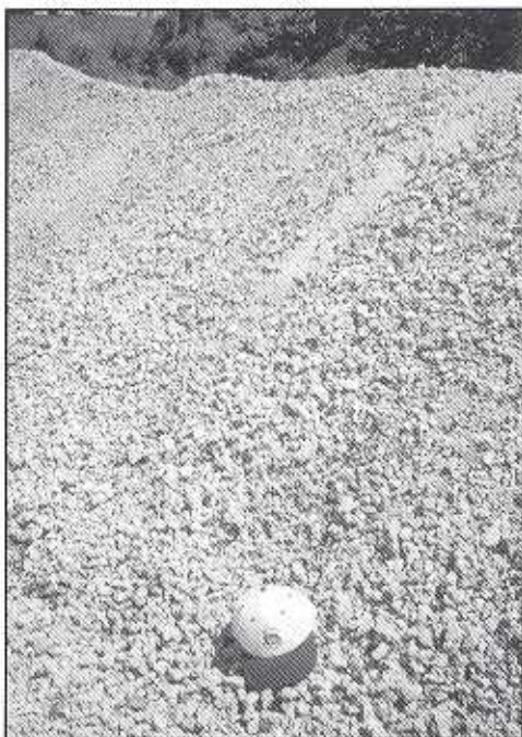
Recycled pavement, crushed to Gradation #14, to be used as subbase for new pavement.
